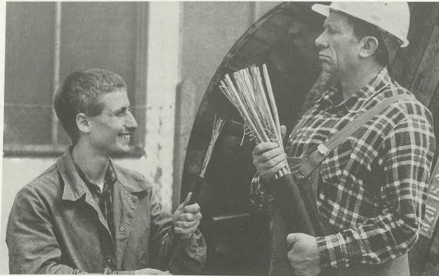
Figure 7.9 The relative sizes of fibre and copper cables
