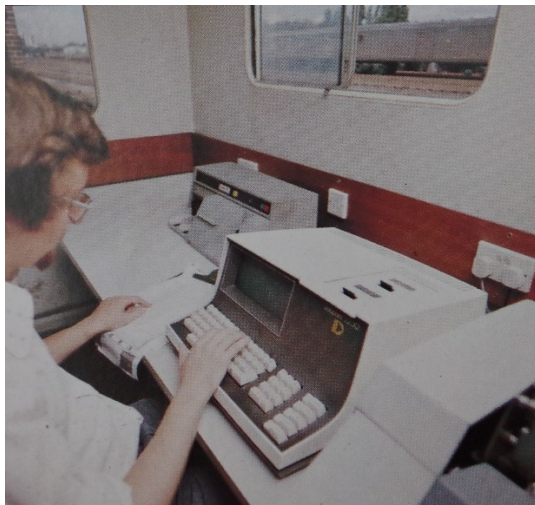
Figure 7. Area Freight Centres used minicomputers to help transmit and receive TOPS information. Note the small CRT screen and two cassette tape drives on top. The purpose built desk conceals the interface equipment in the "tank".
